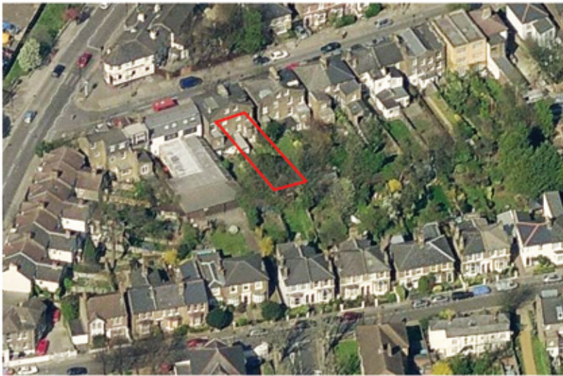
EXISTING AERIAL VIEW
